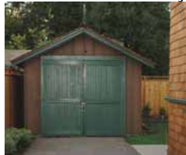
The newly renovated garage, 2005.
